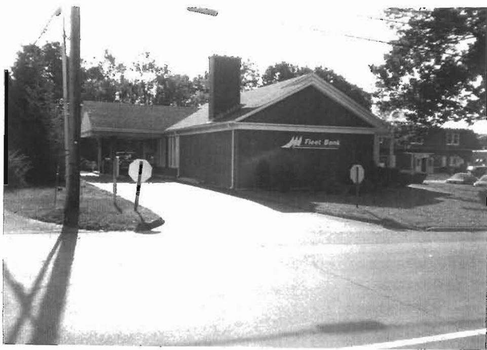
Front view of subject property from Dog Lane
