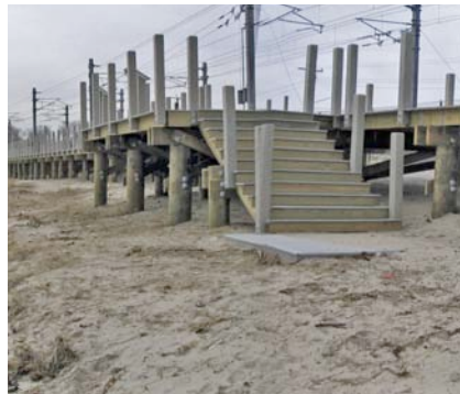
The wooden steps to the Boardwalk in Niantic are shown here in 2004 (L) and in 2007 (R). Engineers anticipated the seasonal rise and fall of the beach by including deep-rooted supports into the design of the lowest steps. Unfortunately, the steps now are undermined and exposed year-round.
