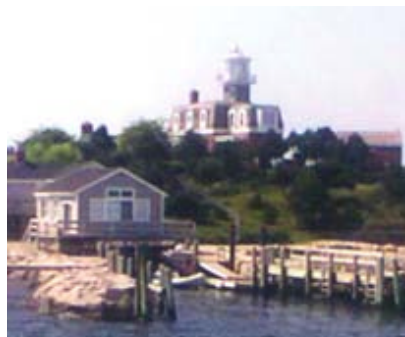
North Dumpling Lighthouse
